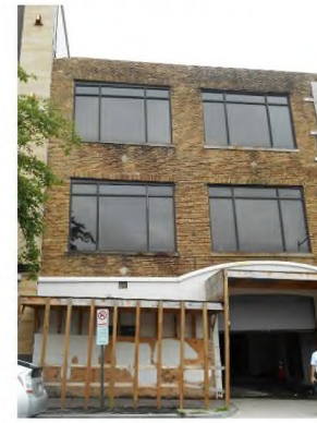
VIEW E: NE CORNER FROM KALORAMA RD
