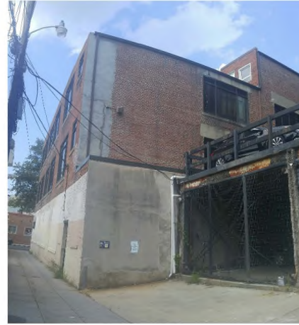
VIEW B: SW CORNER FROM THE ALLEY LOOKING NORTH
