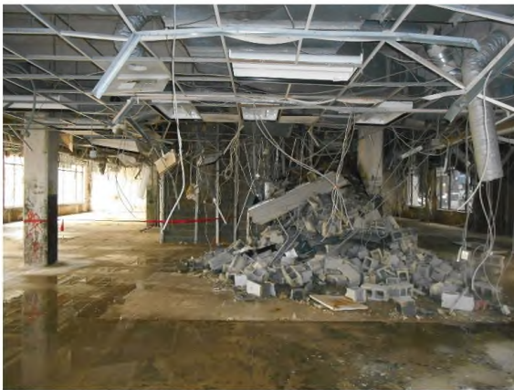
VIEW C: EXISTING CONDITIONS OF THIRD FLOOR FROM WEST LOOKING EAST
