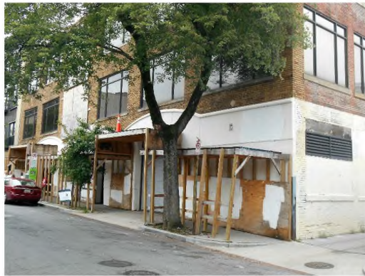
VIEW C: NW CORNER FROM KALORAMA RD NW LOOKING SOUTH EAST
