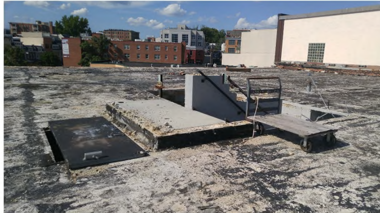
VIEW D: EXISTING ROOF
